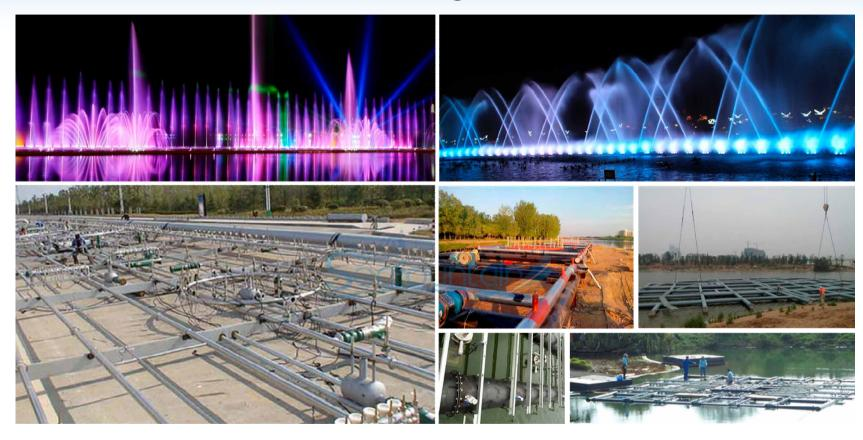
Lake Floating Fountain are named from the installation form. Different from the normal fountain that installed on the water pond or underground, the Floating Water Fountains are installed on the floating platform, which could rise or drop with the water level changes, so the fountain working would not be affected by seasonal water level difference.
